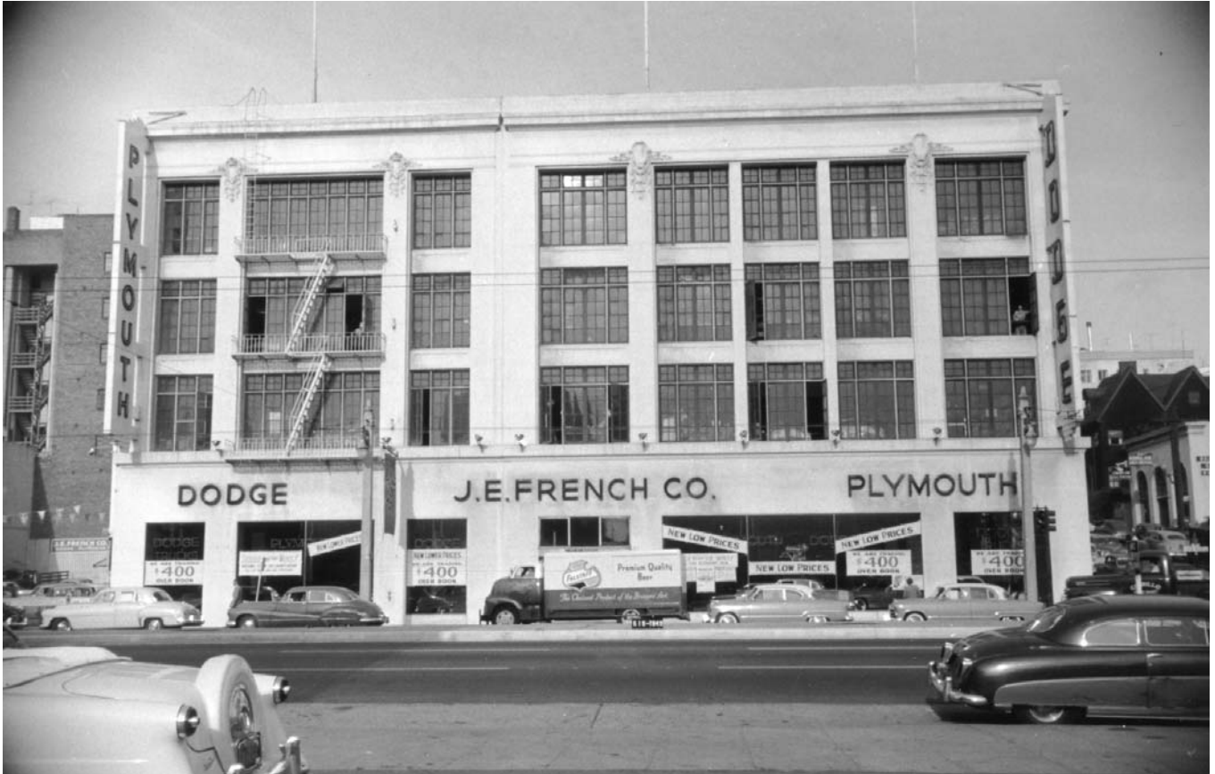
This building in the 1950s. The three bays to the south (at left) constitute the addition of 1926. The first story has already been altered, and is very similar in character to how it is today. The ornament atop the piers is still in place in this photo. From the SF Public Library, Assessor's negatives.
