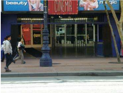
Detail of primary entrance. 103_3830.JPG 3/3/2011
