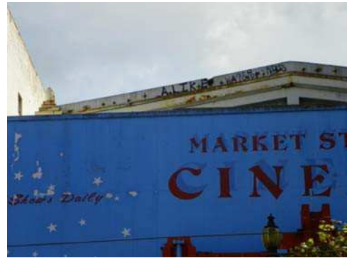
Detail of roofline. 103_3829.JPG 3/3/2011
