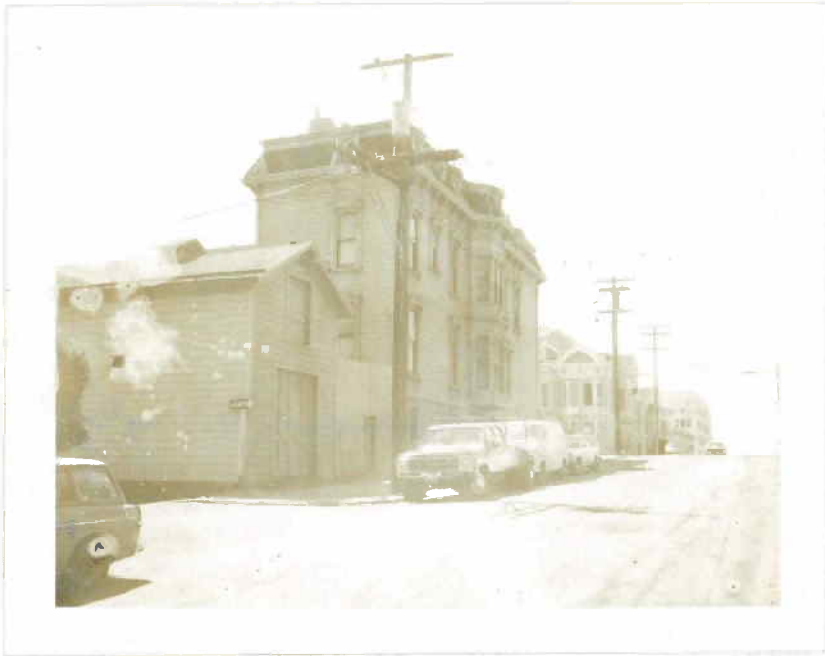
Rear view of 198 Haight showing Carriage House
