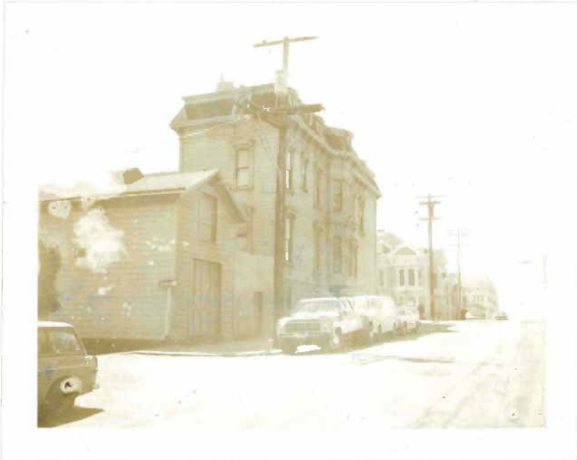
Rear view of 198 Haight showing Carriage House
