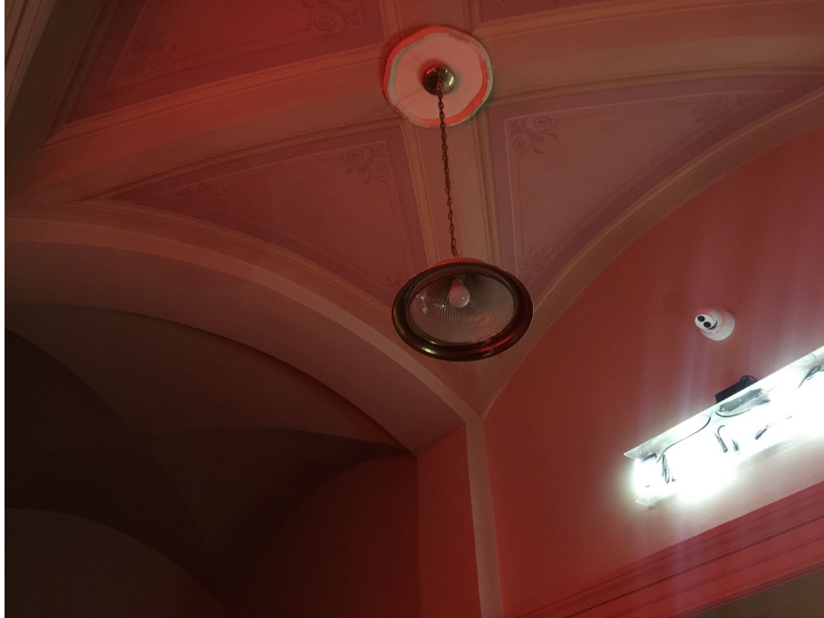
Ceiling and light fixture of the foyer, view northwest.
