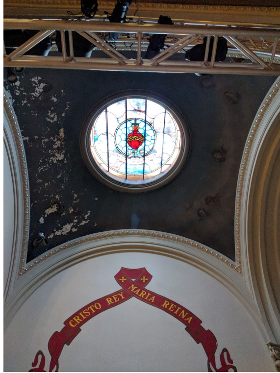
Stained glass on ceiling along western side aisle, view west.
