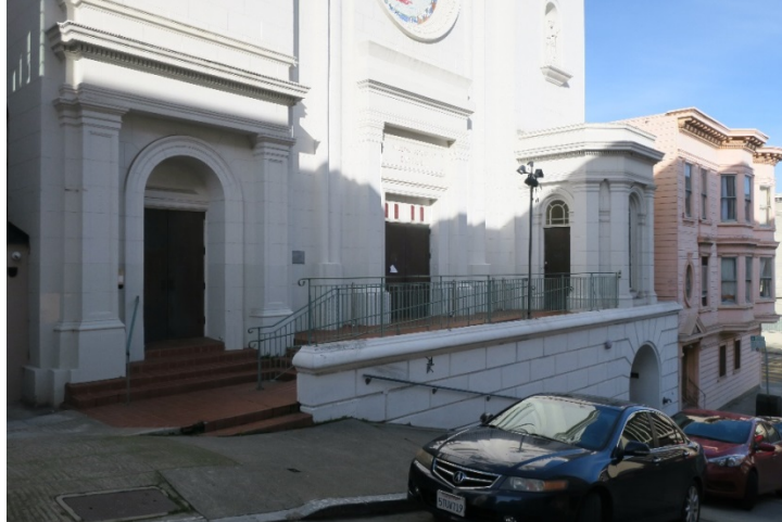
Primary façade entries, with projecting one-story bay east of central entry. (Page & Turnbull)
