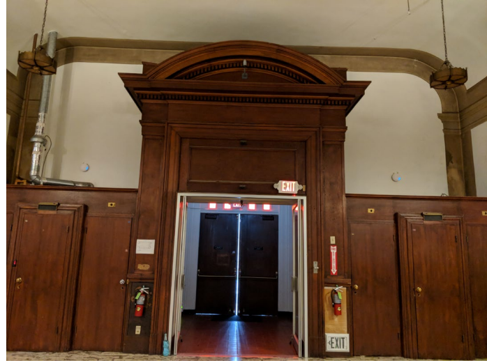
Detail of woodwork at narthex wall.
